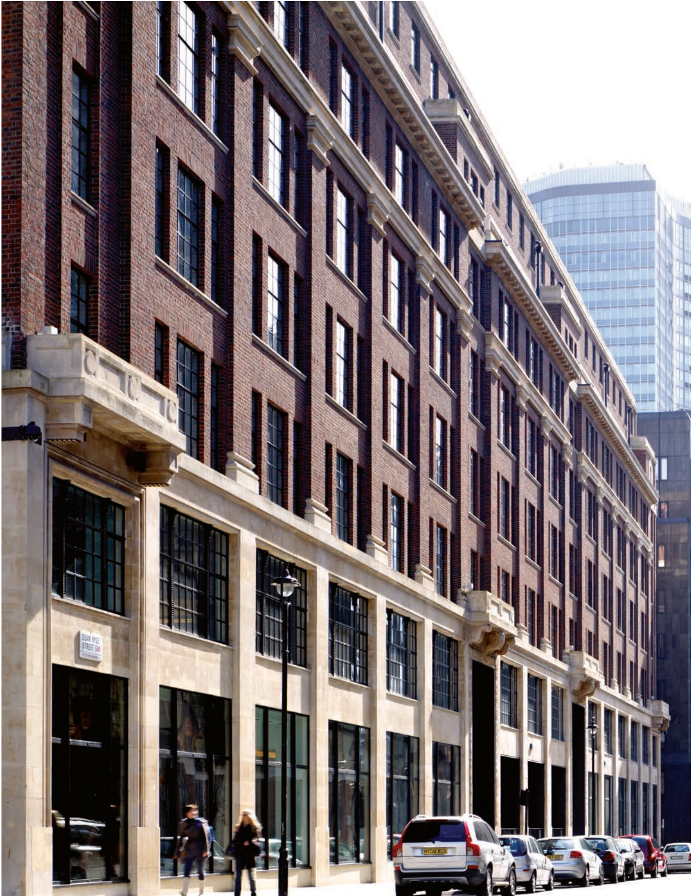
View looking south of the Dean Ryle street facade
