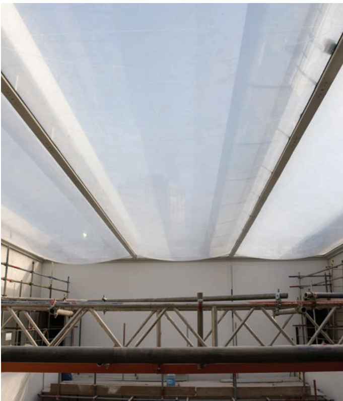
ETFE roof during construction
