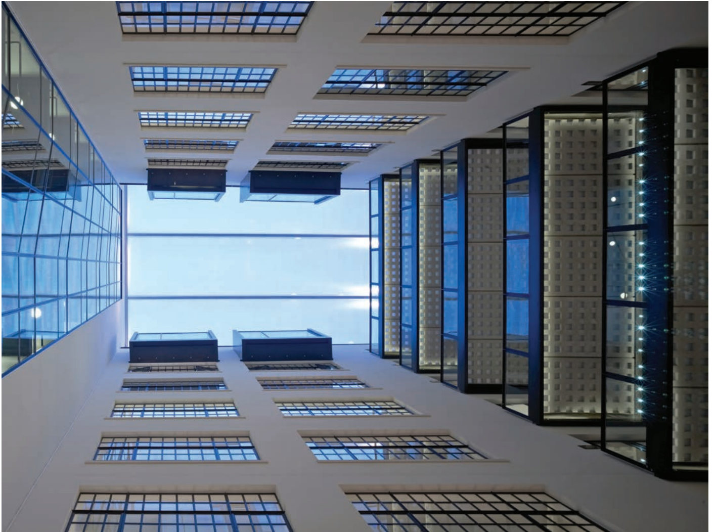
View of the atrium and the ETFE roof
