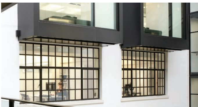
View into offices, from bridge
