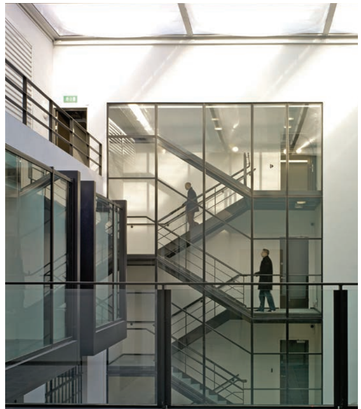
ETFE roof, completed building
