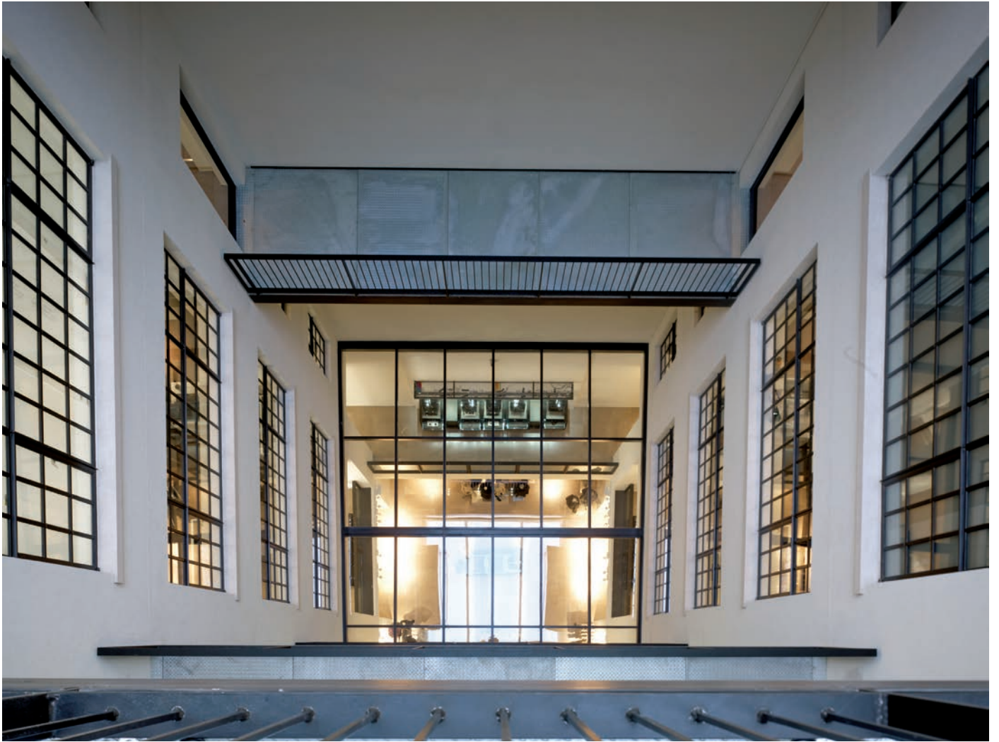
View of the lightwell and the glazed roof to the ground and lower ground office
