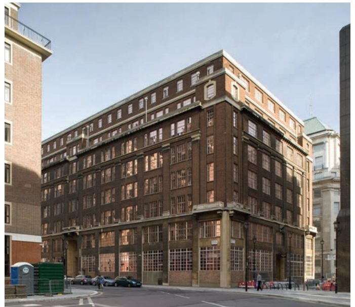
Views of the existing building showing entrance to Horseferry Road
