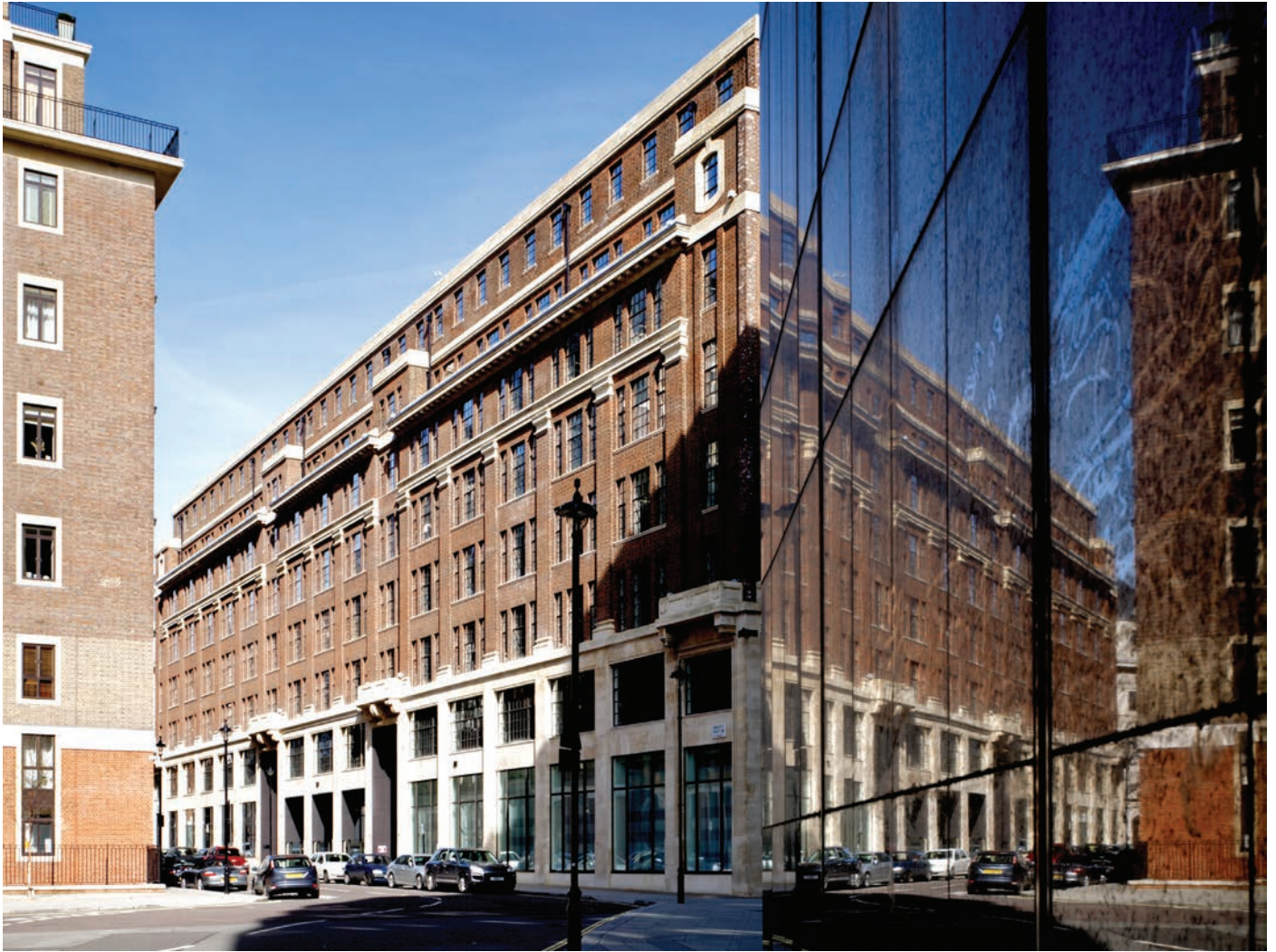
View from Dean Ryle Street looking north
