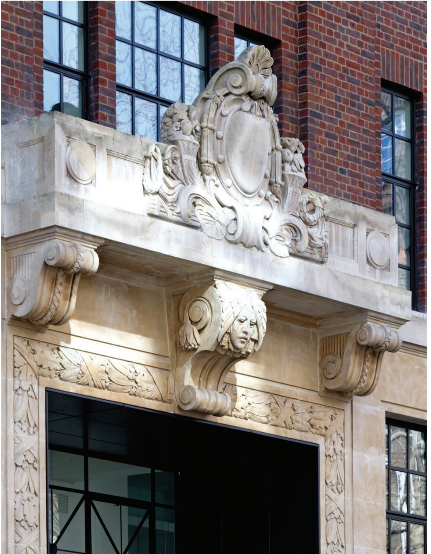
Restored view of sandstone detail around the buildings portals
