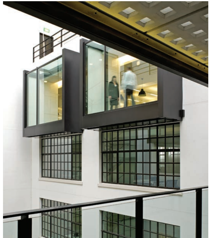
View of one of the higher level pop outs, completed building
