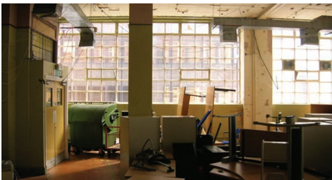
View of existing office floor
