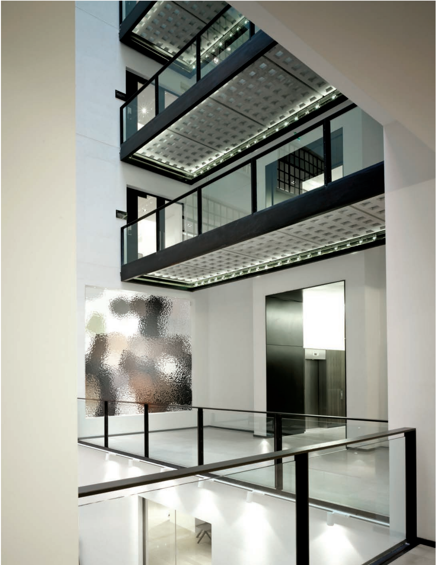
View across atrium of the pre-cast bridges in front of the central core
